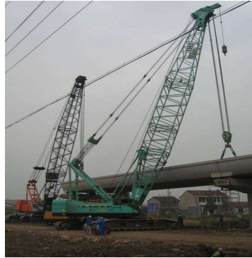
Figure 1: Placing full precast span (with crane)
