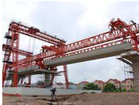
Figure 2: Placing full precast span (with launching girder)
